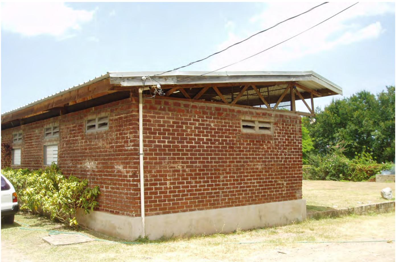
*Building at the Jamaica Bauxite Institute with bricks made from bauxite residue.*
