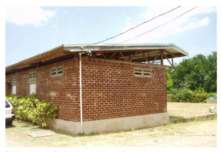
Building at the Jamaica Bauxite Institute with bricks made from bauxite residue.
