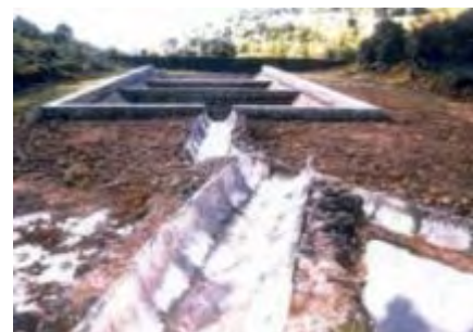
Figure 7.2 Silt dams in series and settling of silt in tanks at Hindalco Durgmanwadi, India
