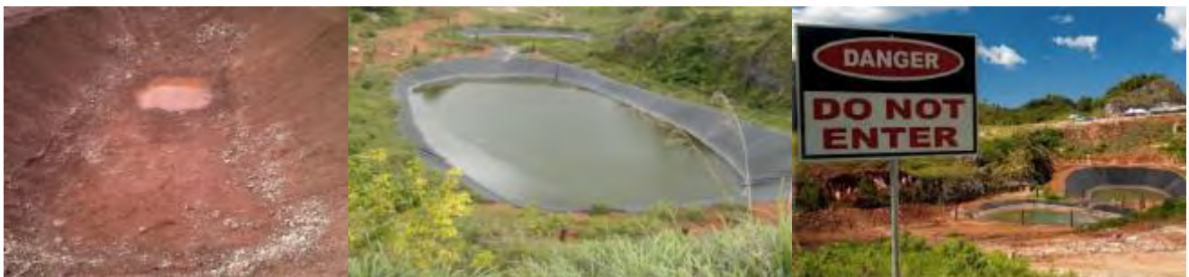
Figure 7.6. Bauxite pit converted to 5 million gallon capacity pond, Tobolski, St Ann, Jamaica
