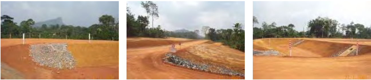
Figure 7.23 Combined temporary and permanent erosion control at Alufer Bel Air, Guinea
