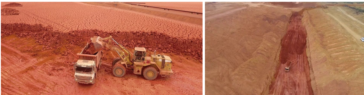
Figure 56: Removal of dry tailings from RP1 dam and disposal at the mine pits
